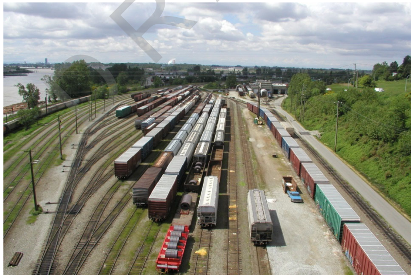
Aerial view of Trapp Yard looking towards Burnaby
